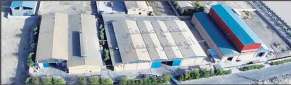
Peyman Aluminium Industrial Complex
