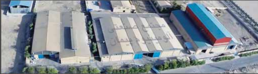
Peyman Aluminium Industrial Complex
