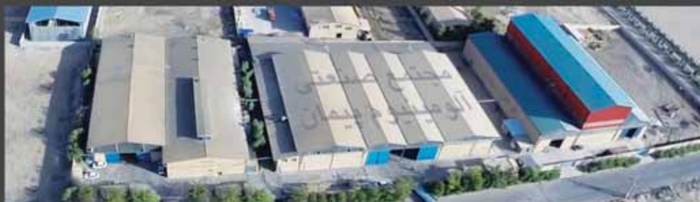
Peyman Aluminium Industrial Complex
