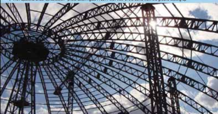
The Aquatoria under construction - photo taken August 7, 2011 with view of the dome from the ground looking up
