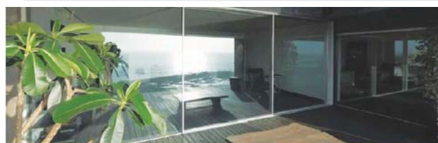
fig. 16 - PanoramAH! Movable Glass Wall Systems installed in Mumbai
